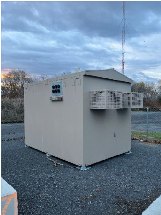
Photo 1. Example of CMT hut to be installed on proposed sites. Structure measures approx. 8 by 12 feet.
