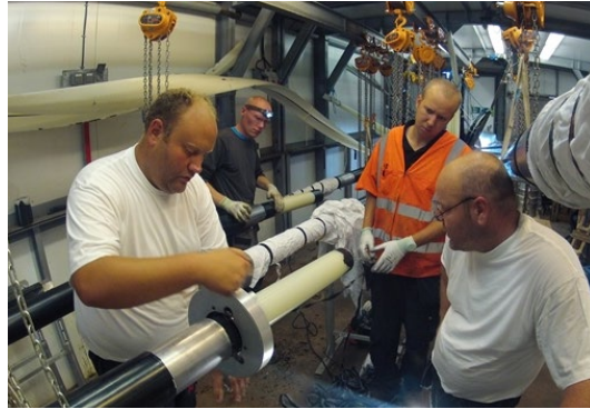
Figure 3. Preparation of Cable Ends Prior to Installation of Splice in Progress
