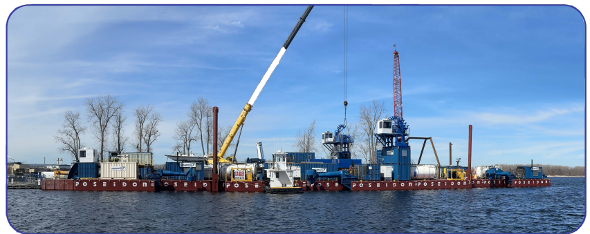
Main Cable Installation Vessel
