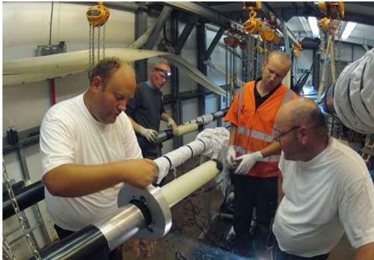
Figure 5. Preparation of Cable Ends Prior to Installation of Splice in Progress
