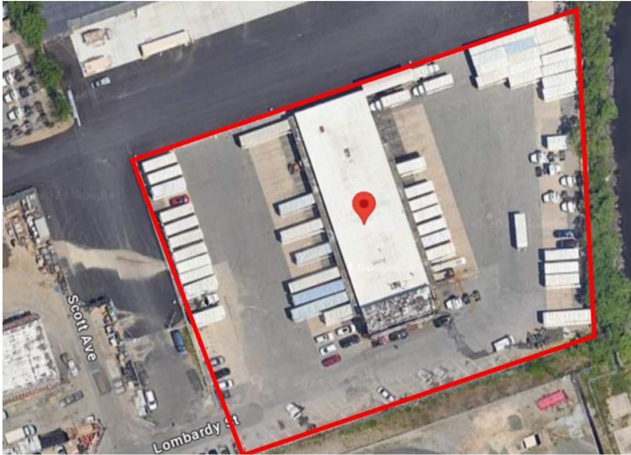
Yard No. 2 – Old Dominion Freight (Leased by E-J Electric) 295 Lombardy Street, Brooklyn, NY 11222
