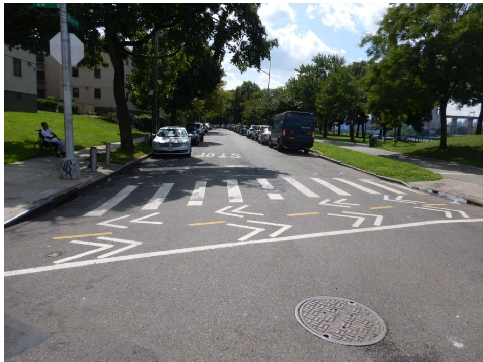
Figure 8. Astoria Rainey cable route on Shore Boulevard at its junction with 20 th Avenue. The greenspace on the right is Ralph Demarco Park. View facing southwest.
