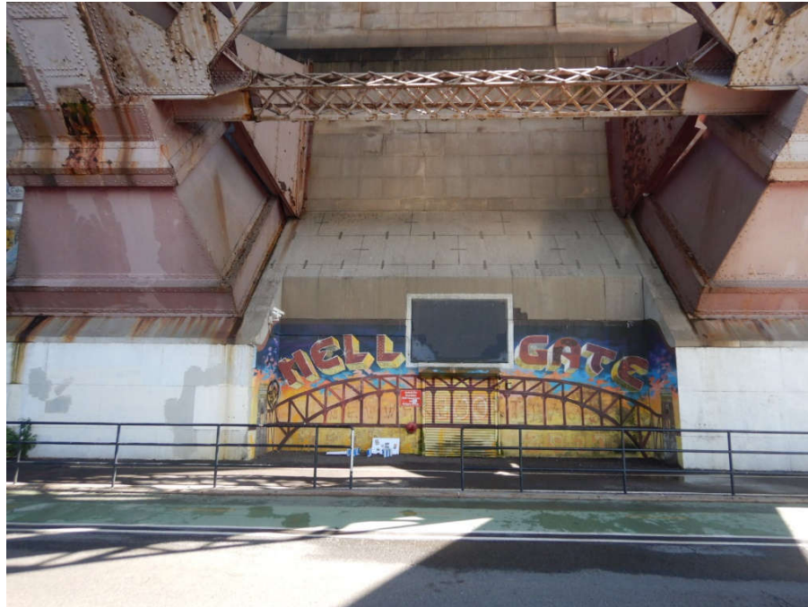
Figure 12. Southeastern tower or base of the Hell Gate Bridge (08101.000043), a 1917 railroad bridge that crosses the East River from Randalls Island to Queens. The Astoria-Rainey cable route will be in Shore Boulevard, in the foreground (near the bottom) of this photo. View facing southeast.
