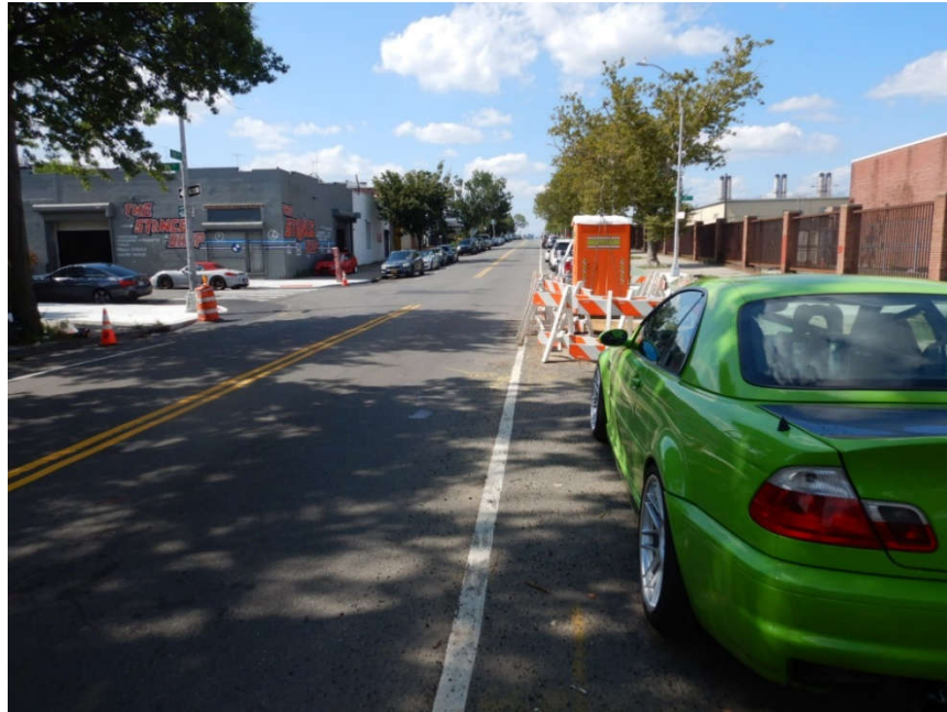
Figure 9. 20 th Avenue near 29 th Street. View facing northwest.
