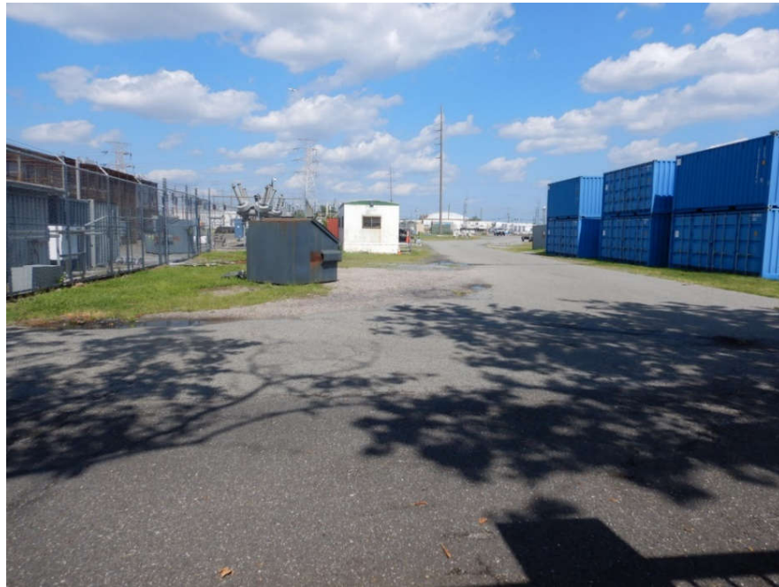
Figure 10. Spur of 19 th Avenue, the route the Astoria Rainey cable will take to reach the Astoria Annex substation. View facing northeast.
