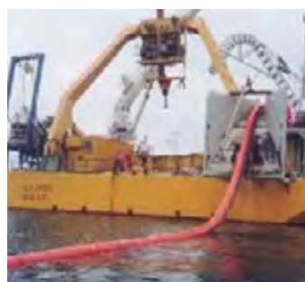
3. The HVAC cable and SeaSerpent being deployed at Havelet Bay.
