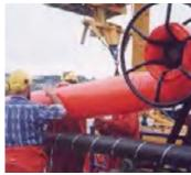
SeaSerpent being attached to the HVAC cable showing Seaflex manual brake RDS.
