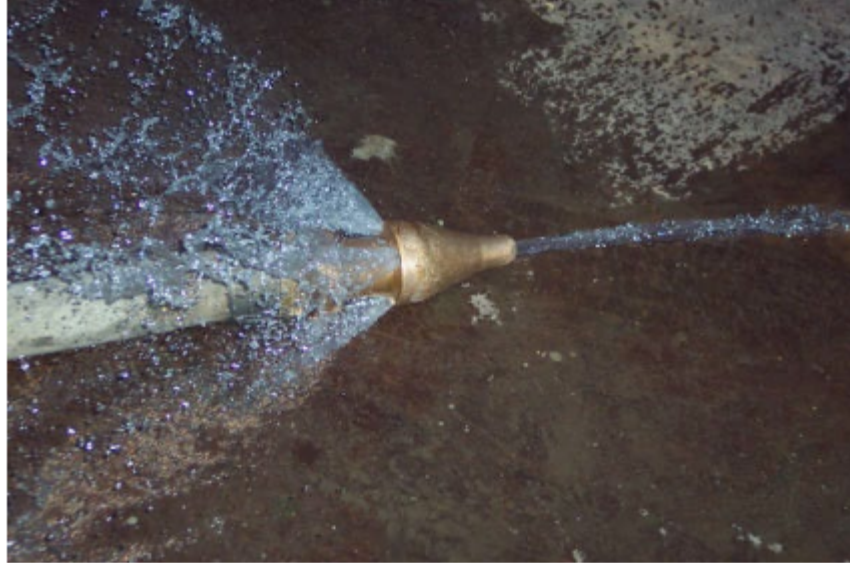
Figure 20-'Navy type' reactionless jet nozzle (diver operated)
