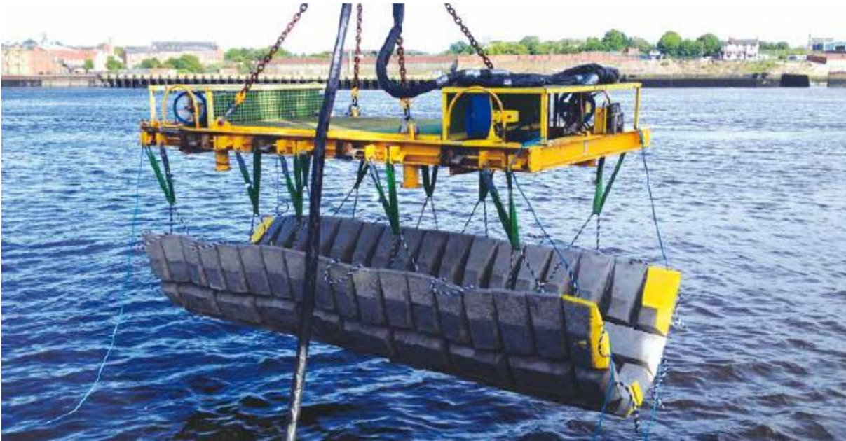
Figure 7 Indicative ROV Mattress Deployment Frame
