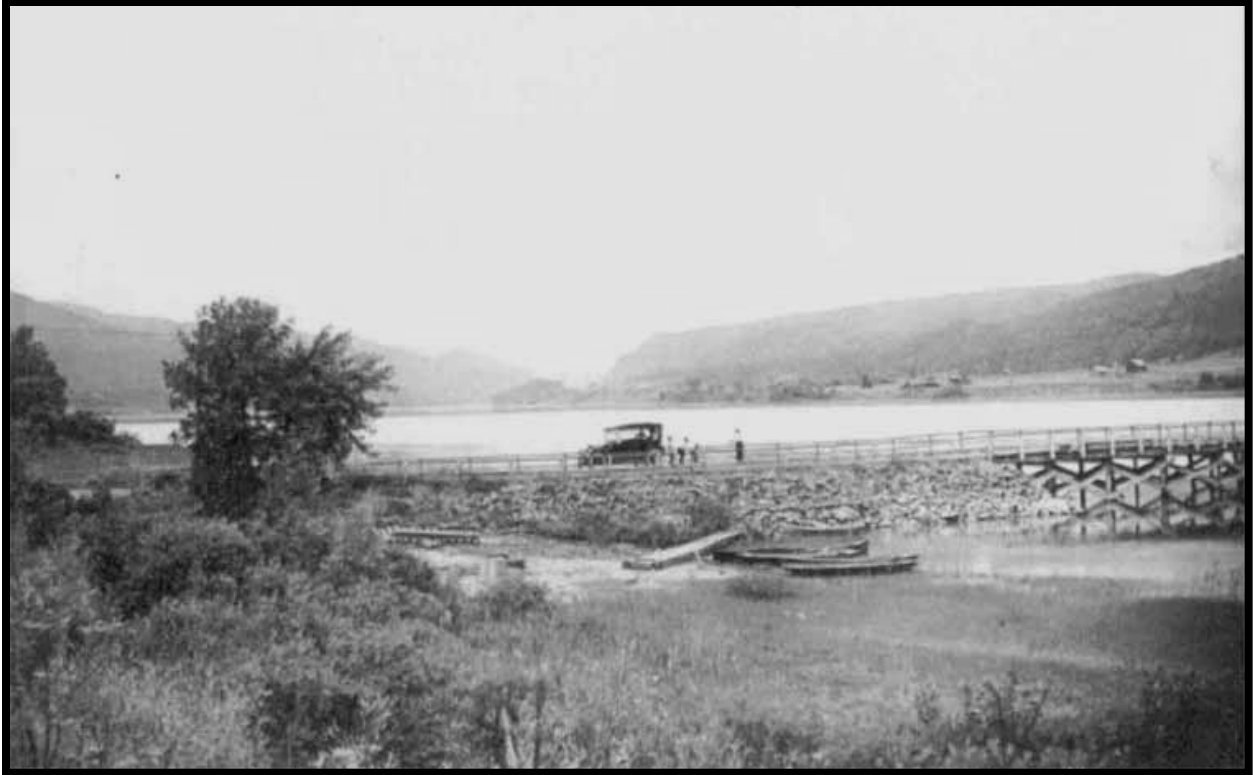
Figure 6-4. Photo showing the west end of the 1913 bridge looking south (courtesy of the Historical Society of Whitehall).
