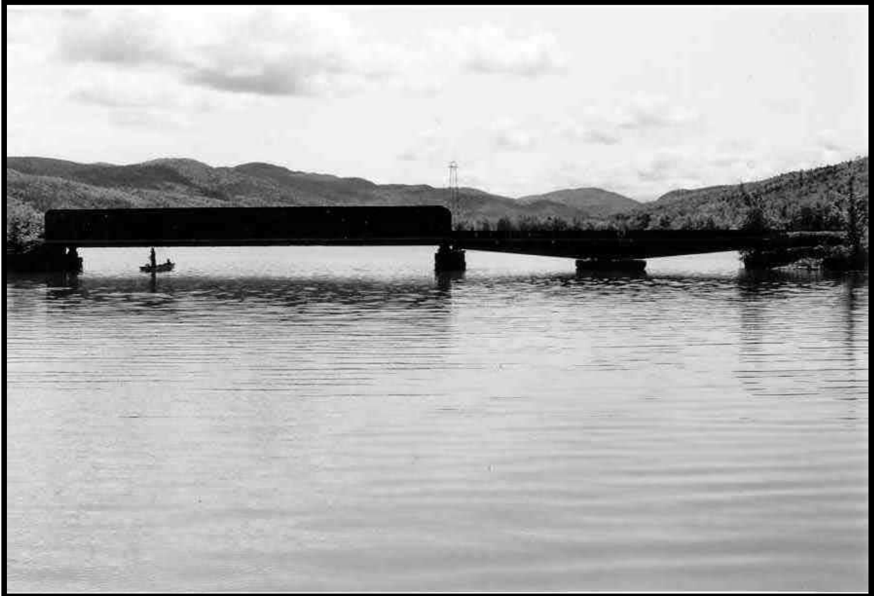
Figure 6-2. Photo of the original railroad drawbridge crossing South Bay looking northerly (by A. Peter Barrannco).
