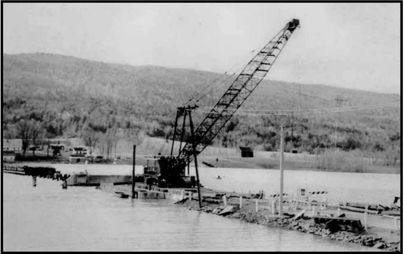
Figure 6-5. Photo taken circa 1972 of the removal of the 1932 bridge, looking northwest toward Dresden shore (courtesy of the Historical Society of Whitehall).
