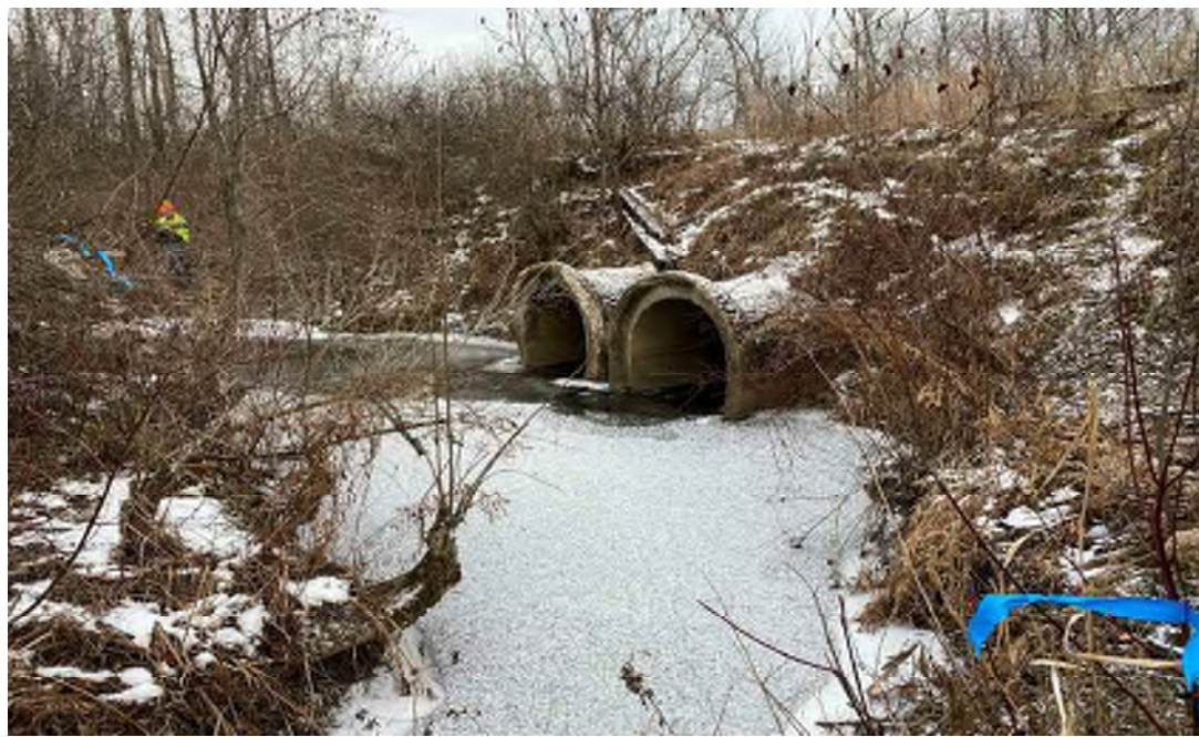
Stream C-R-S1/G-R-S-K - downstream
