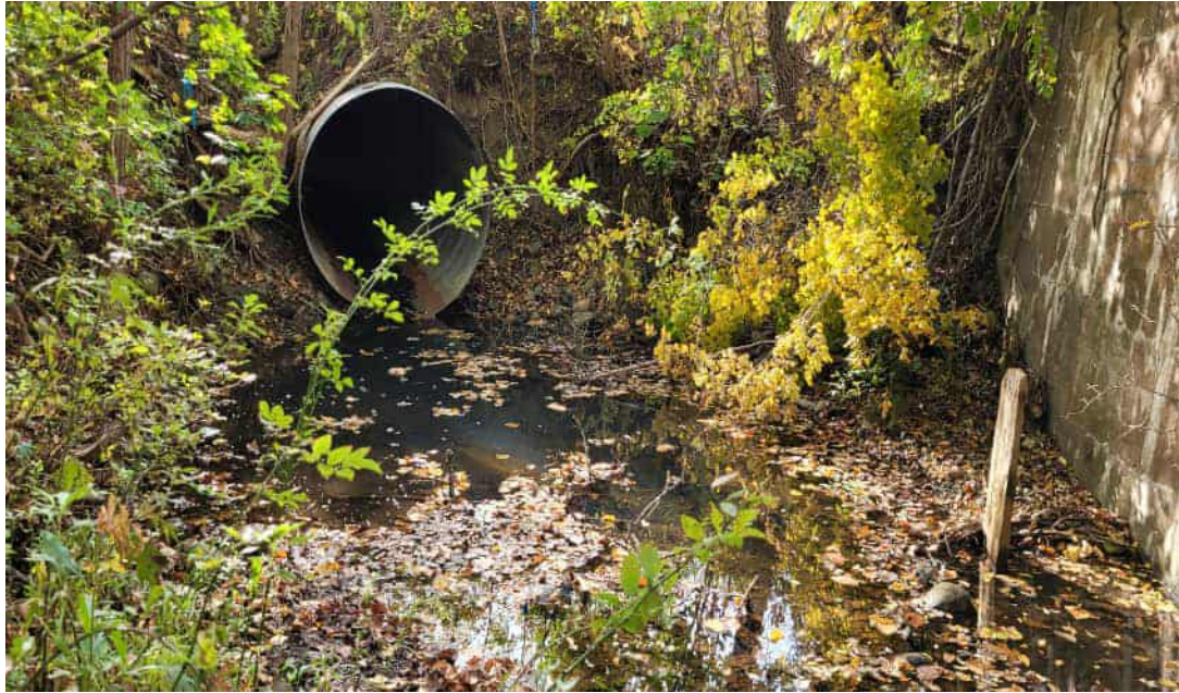
Stream P5-S6 - upstream Lat: 42.599306 Long: -73.886726
