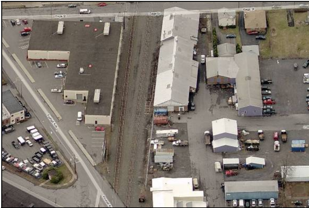
View of Large Buildings Immediately Adjacent to Railroad Corridor in Kingston
