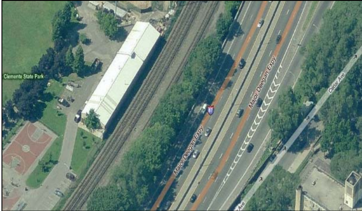
View of Building Immediately adjacent to Railroad along Harlem River
